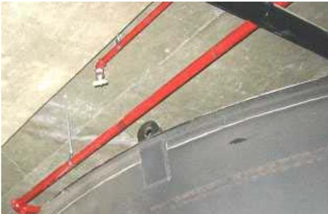
This is a consideration that the designer always has to keep in mind as it is an important part of what is considered good design and engineering practices. A subsequent discharge test proved that the design covered every area adequately with compressed air foam.
